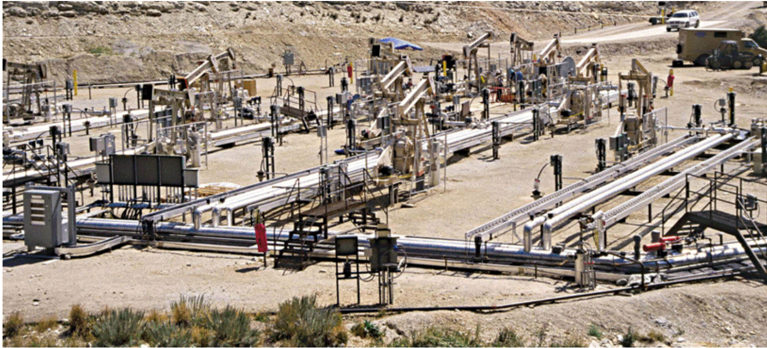
Shell Oil plant, Piceance Basin, Colorado, USA
